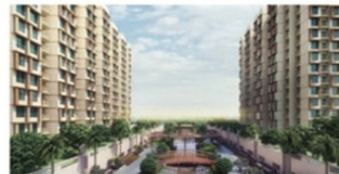
CONSTRUCTION IN FULL SWING
